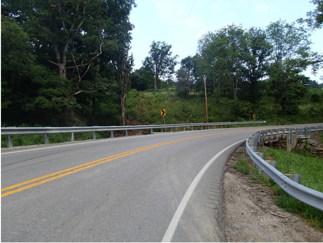
Figure 4-17. View of General Project Area: Curve and Bridge on US 460. Looking Northwest.
